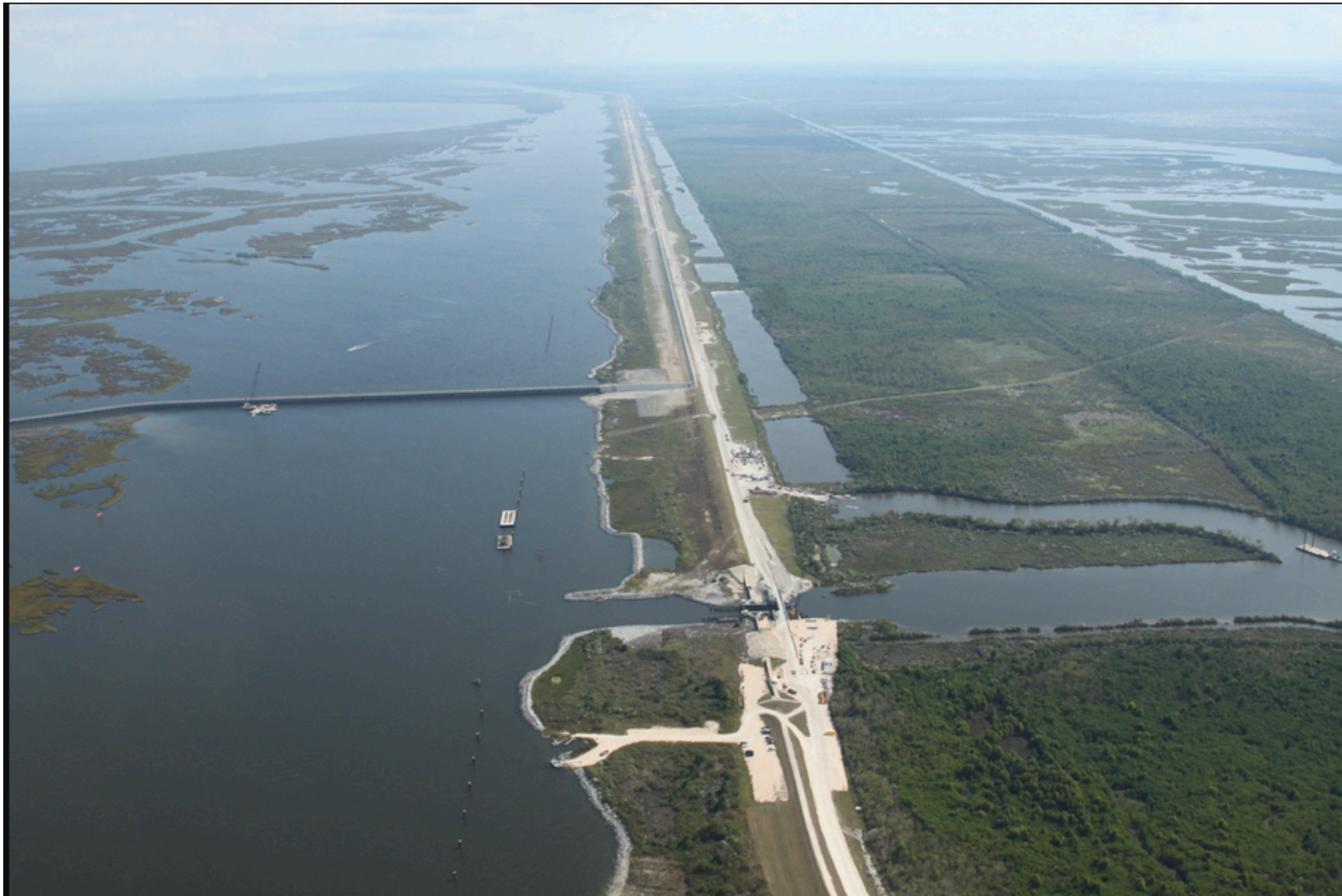
Floodwall construction at St. Bernard Parish
